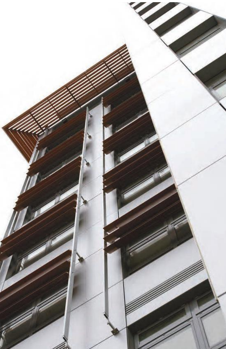
Trafalgar House United Kingdom QuadroClad
