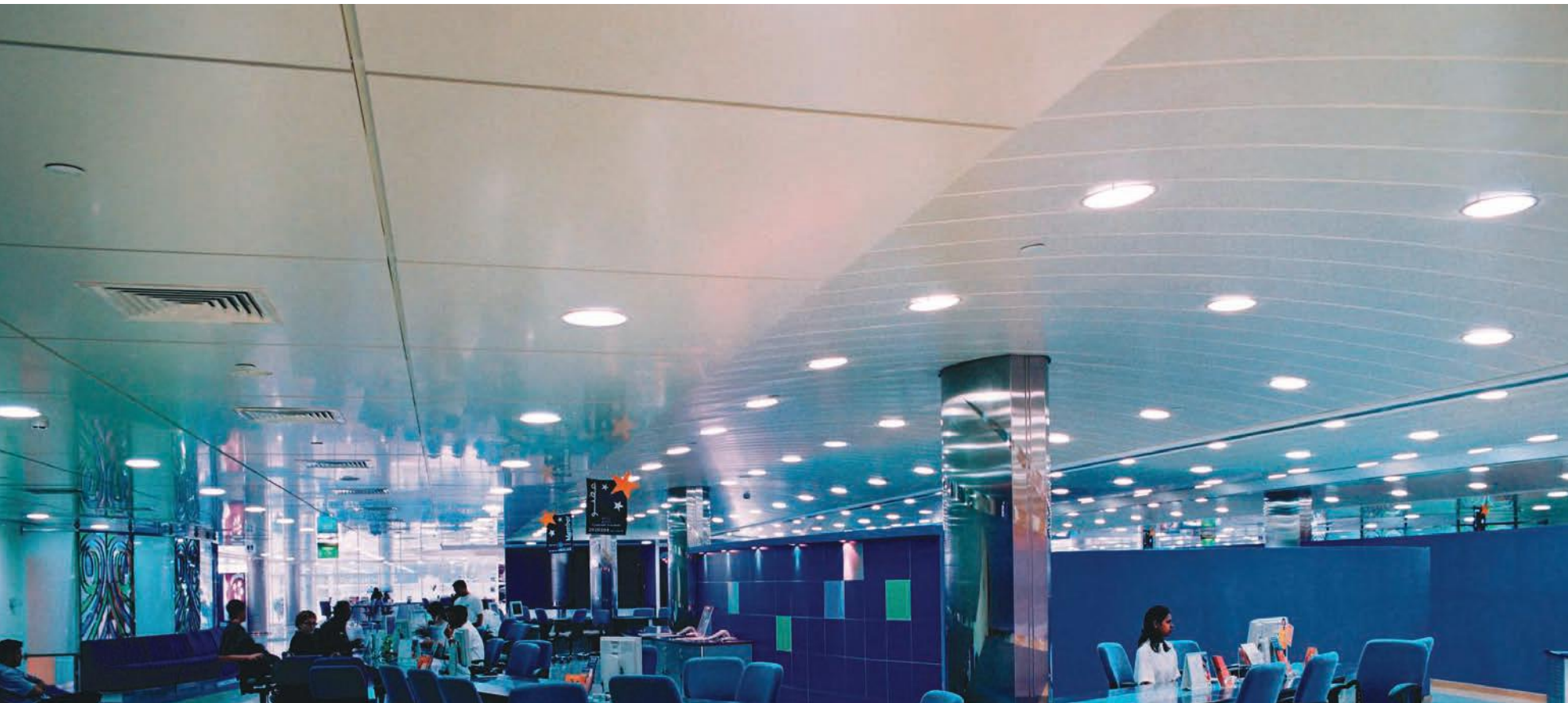
Dnata Airline, Dubai Lay In Tile Ceiling
