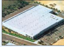
Hunter Douglas Fabrication, Poway (CA), U.S.A.
