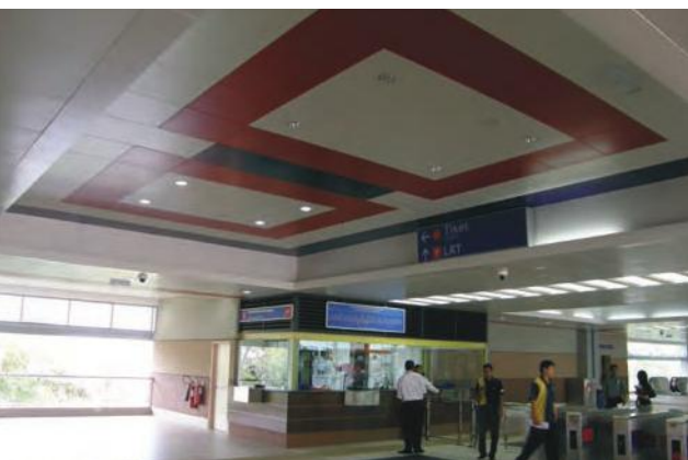
LRT station@Sri Rampai, Kuala Lumpur, Malaysia Clip-in Tile ceiling
