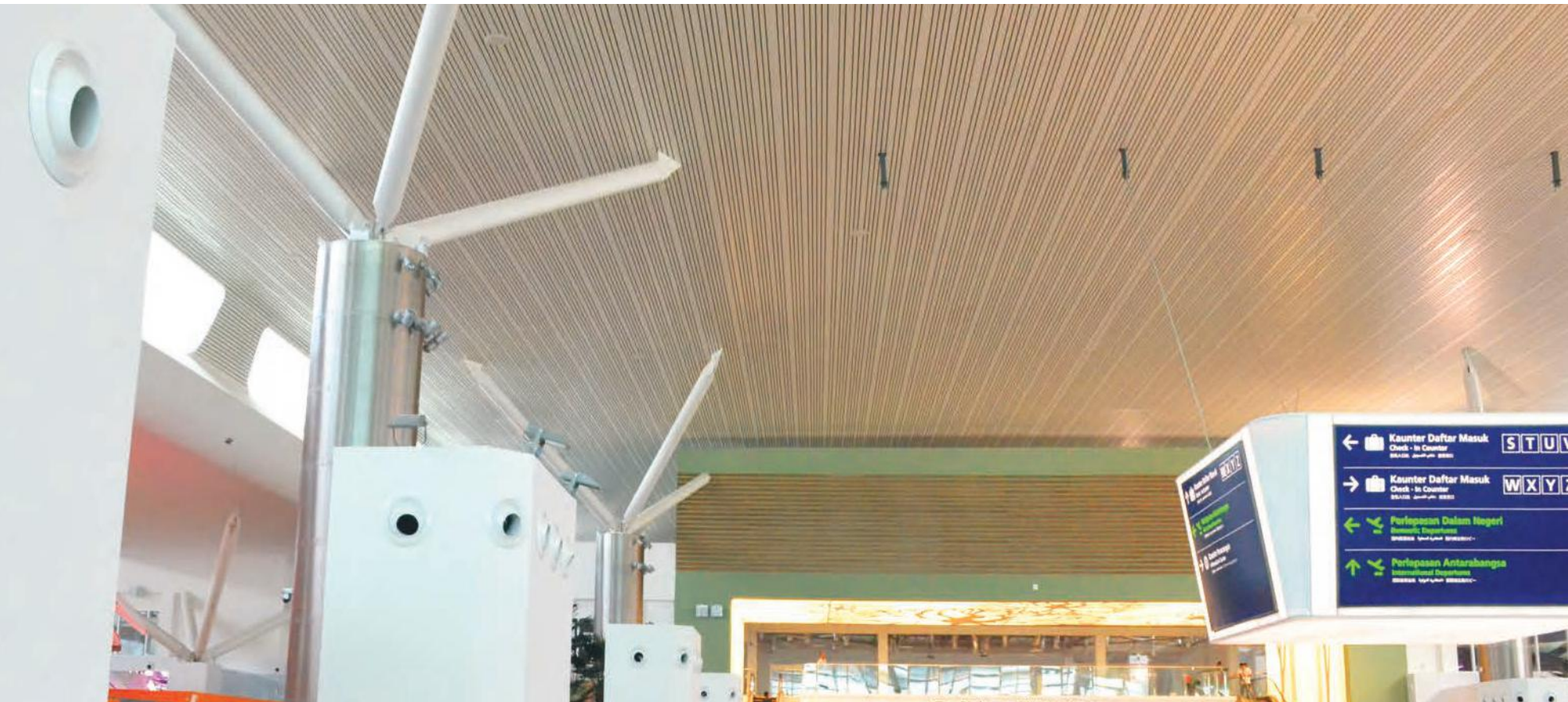
KLIA2 Malaysia Multi B ceiling
