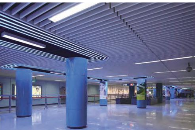
Shanghai Metro Station Line 1 U-Baffle
